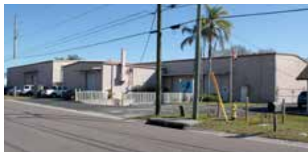
990 Building 2015 to Present
