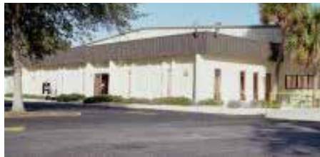
Main Building 1999 to Present
